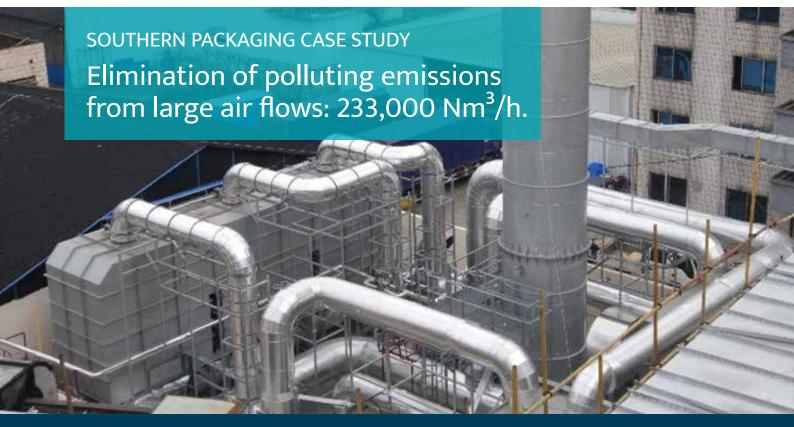
Equipment: RTO + 2 Zeolite rotor-concentrators.
